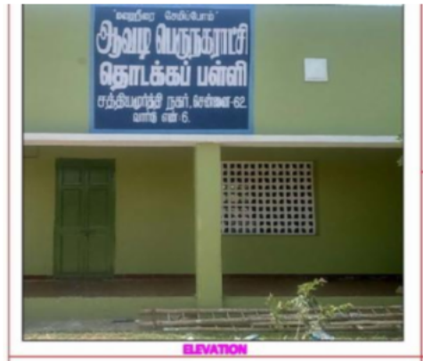
Polling Station Building Front View
