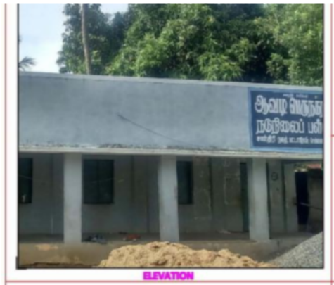
Polling Station Building Front View
