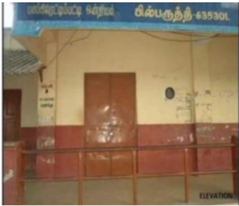
Polling Station Building Front View
