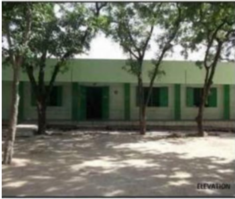
Polling Station Building Front View
