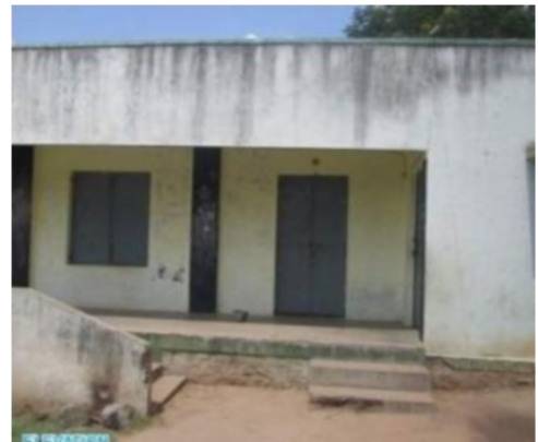
Polling Station Front View
