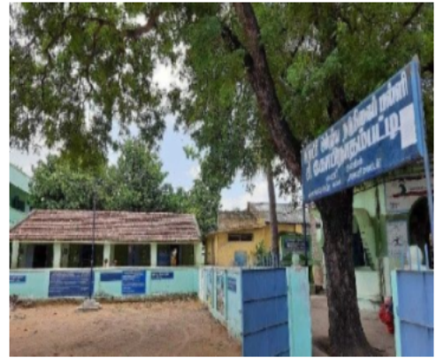
Polling Station Front View
