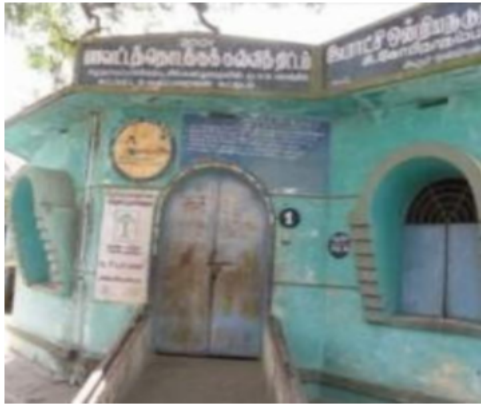
Polling Station Building Front View
