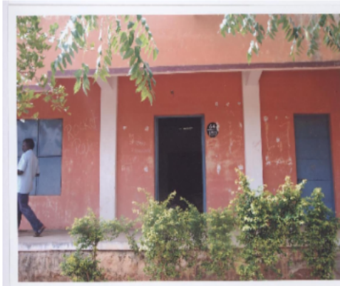
Polling Station Building Front View
