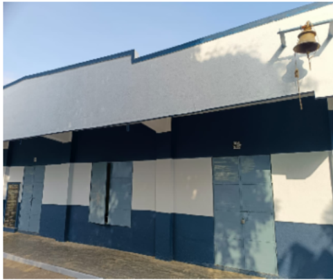
Polling Station Building Front View
