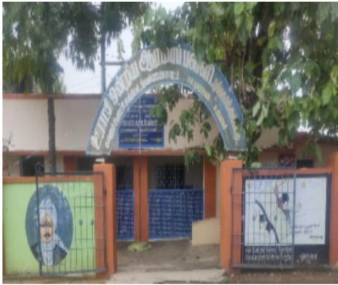
Polling Station Building Front View
