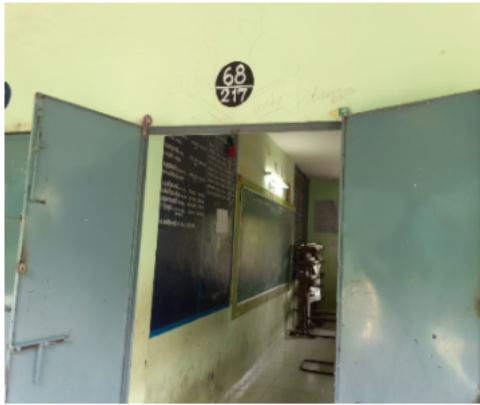
Polling Station Building Front View
