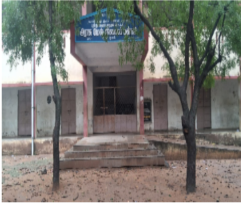
Polling Station Building Front View
