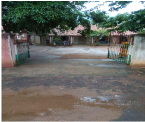
Polling Station Building Front View
