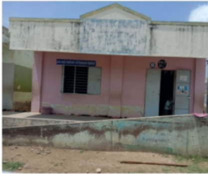
POLLING STATION BUILDING FRONT VIEW
