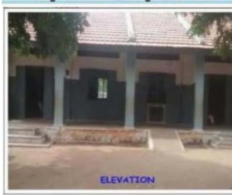
Polling Station Building Front View
