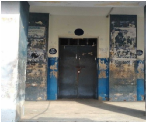
Polling Station Building Front View
