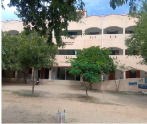
Polling Station Building Front View
