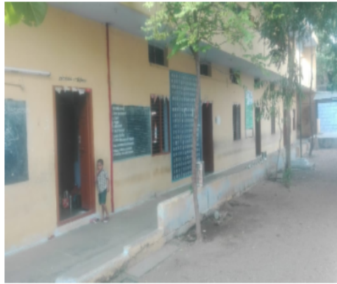
Polling Station Building Front View
