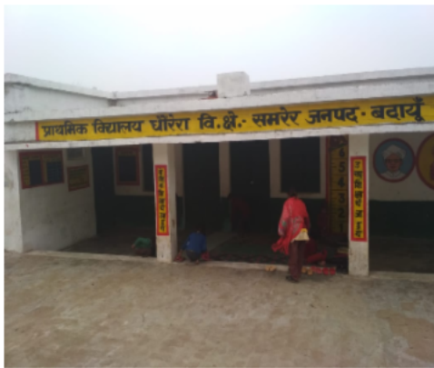
Polling Station Building Front View
