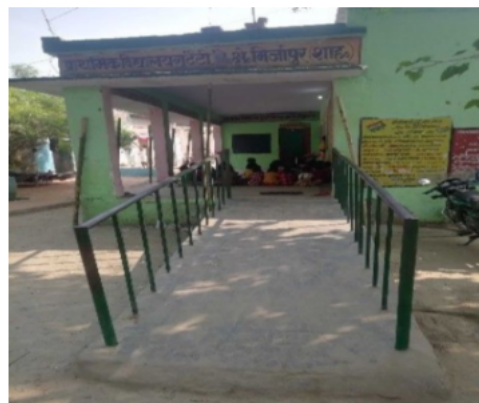
Polling Station Front View
