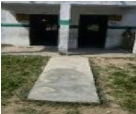
Polling Station Building Front View
