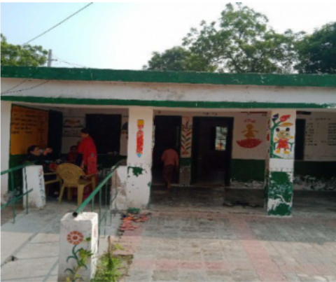
Polling Station Front View
