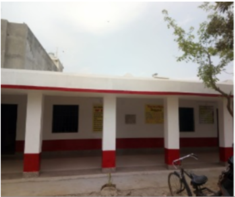
Polling Station Building Front View
