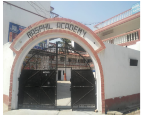
Polling Station Front View
