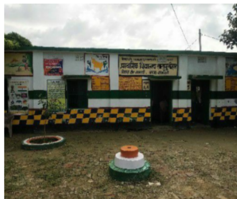
Polling Station Front View
