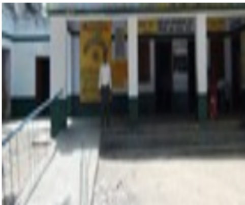
Polling Station Building Front View
