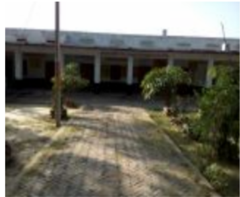
Polling Station Front View
