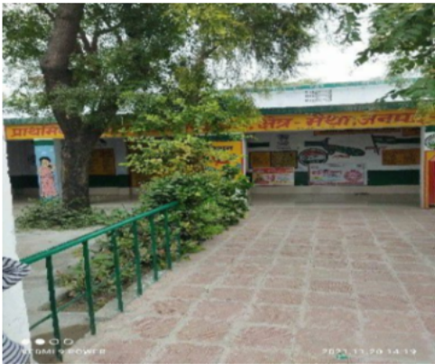
Polling Station Front View
