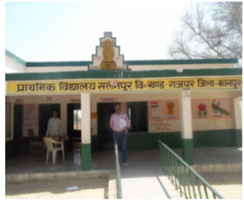
Polling Station Front View
