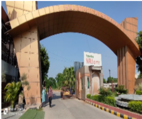
Polling Station Building Front View
