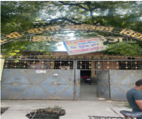
Polling Station Building Front View
