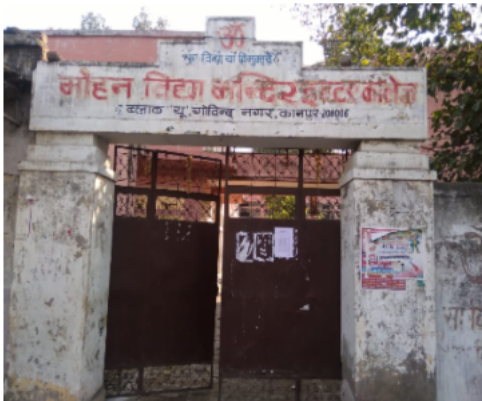
Polling Station Building Front View
