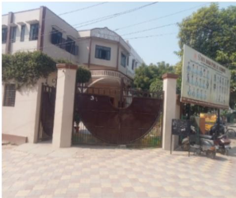
Polling Station Building Front View
