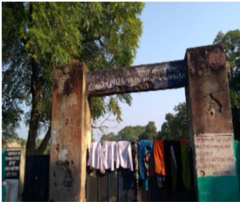
Polling Station Building Front View
