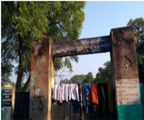
Polling Station Building Front View
