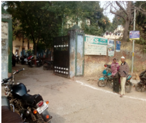
Polling Station Building Front View
