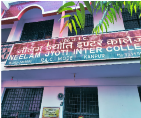
Polling Station Building Front View
