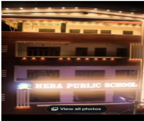
Polling Station Building Front View
