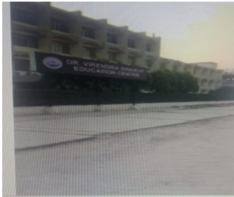
Polling Station Building Front View
