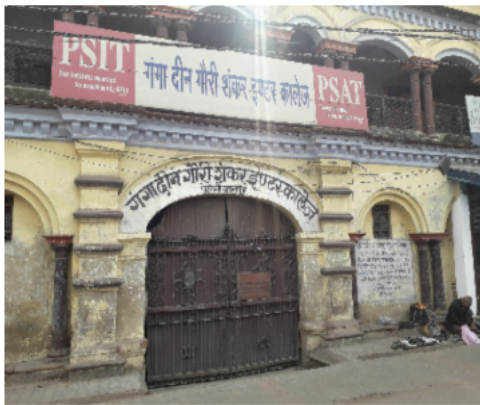
Polling Station Building Front View
