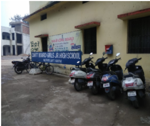
Polling Station Building Front View
