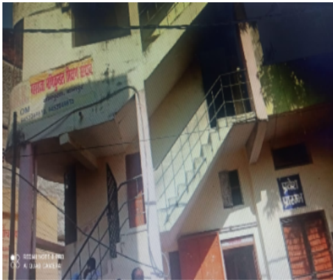
Polling Station Building Front View
