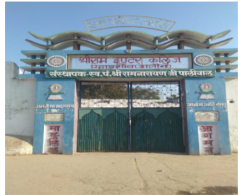
Polling Station Front View
