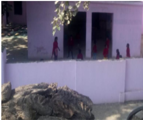
Polling Station Building Front View
