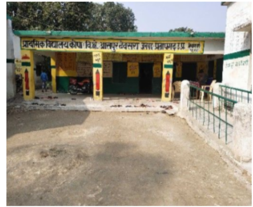
Polling Station Front View
