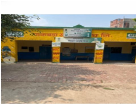
Building Front View
