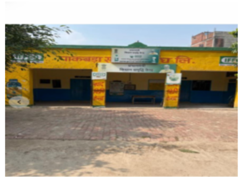
Building Front View
