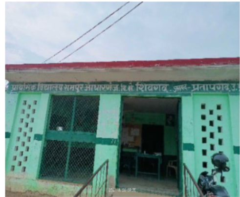
Polling Station Front View
