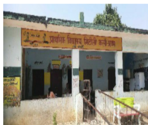
Polling Station Front View
