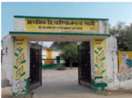
Polling Station Building Front View
