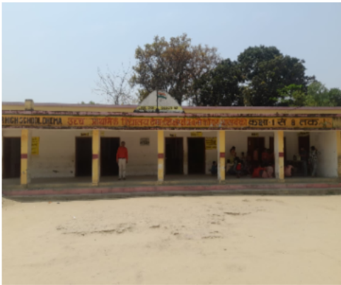
Polling Station Front View
